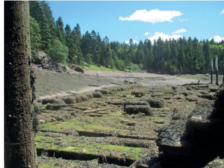
Figure 2. Because of tidal conditions and cold weather exposure, the natural weathering station maintained by the US Army Corps of Engineers at Treat Island, Maine, is useful for assessing the long-term durability of emerging concrete technologies, including alternative binders and blends of portland cement and supplementary and alternative supplementary cementitious materials.
